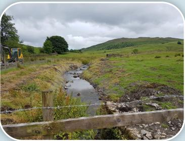
Creation of a new beck for part of a small hydro power scheme. The area within the fence was planted with trees to create improved habitats. Gates and a livestock crossing point were also installed as part of the beck creation project.
