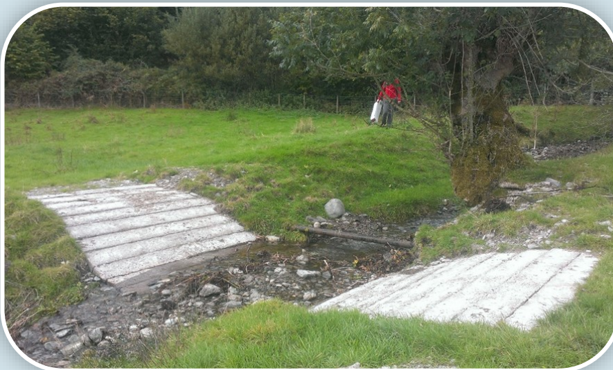
Stream Crossing point installed on a small beck. Prior to installation the banks were steep and eroding from livestock and farm traffic. The banks were regraded to be less steep thereby improving ease of access and vehicle traction whilst reducing sediments entering the beck.
