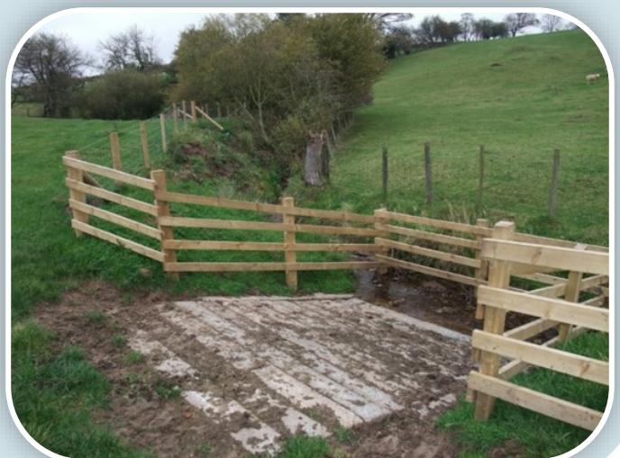
A feeding pad away from the water course. This hard area prevents poaching and loss of sediment and soil from the land.
